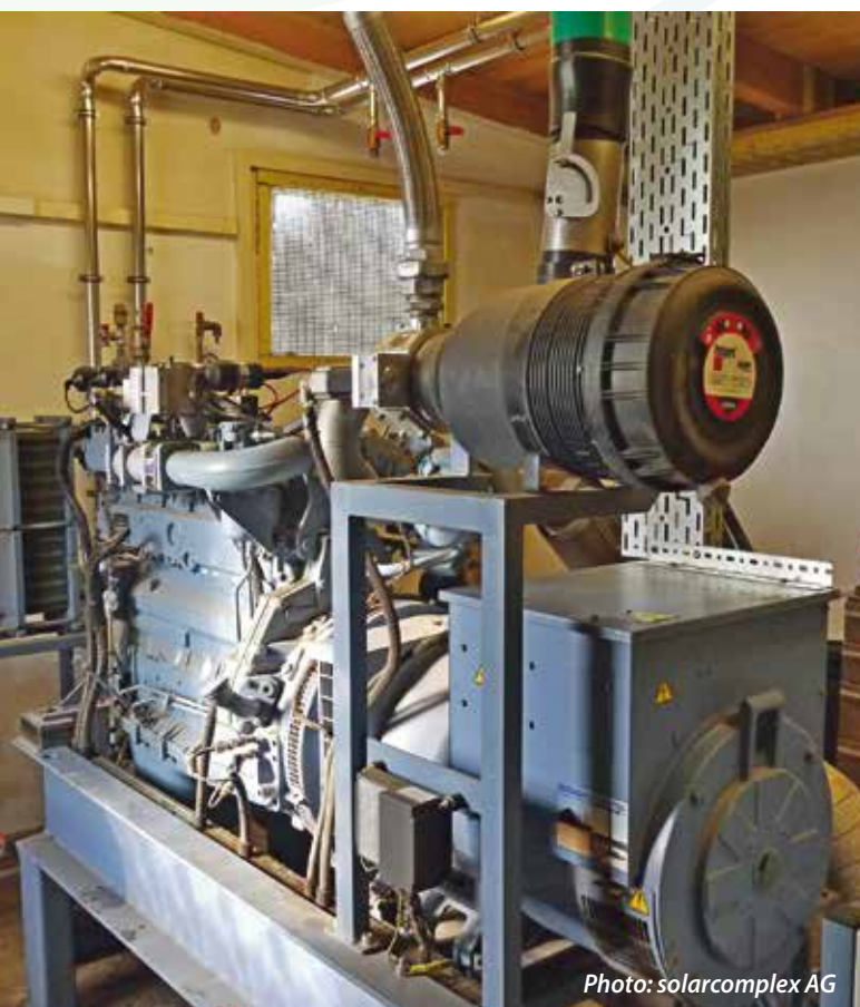
Engine used into the biogas plant
